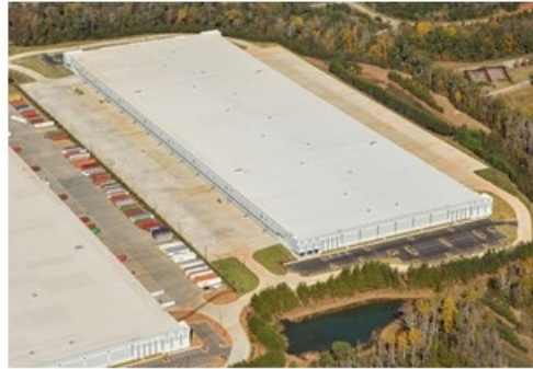
King Mill Distribution Center – Atlanta, Georgia
