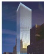
7 World Trade Center • NYC Office Leasing Agent (under construction)
