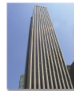
General Motors Building • NYC Office Leasing Agent
